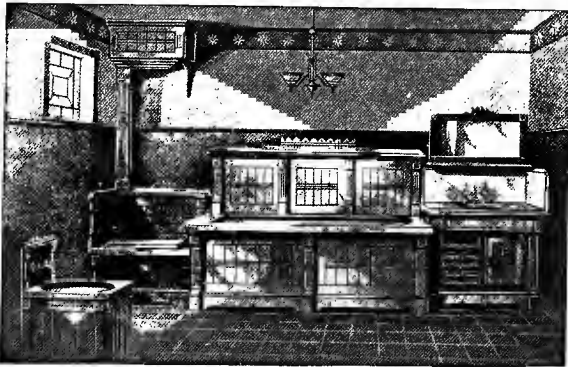
FIG. 11.—Bath room of early 80's. All fixtures are enclosed.
