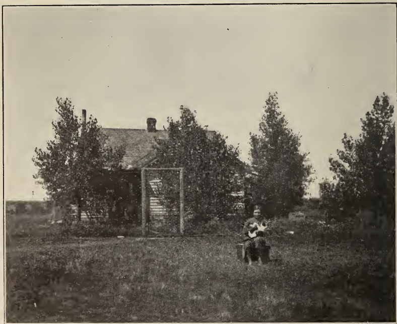
RESIDENCE OF JOHN SARVIS, HYDE COUNTY.
