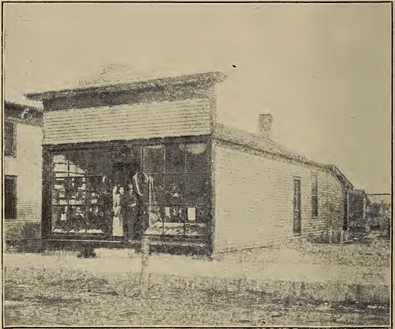
HARNESS SHOP AND STORE BUILDING OF A. DERCK ON IOWA AVENUE
