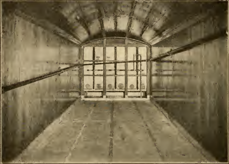
Fig. 1. Interior of milk car cooled by cold pure air
