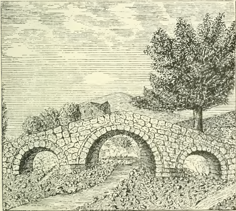
Fig. 74.—ROMAN BRIDGE NEAR MOSTAR.
