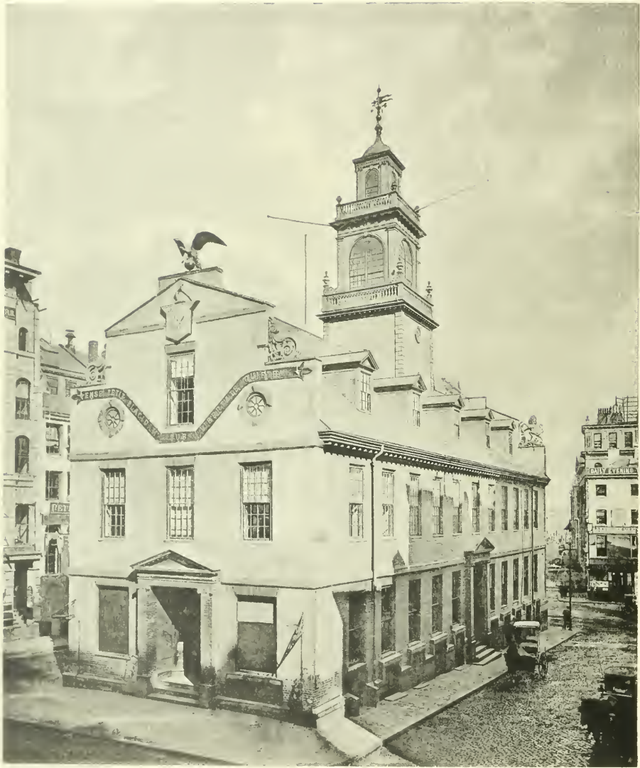
OLD STATE HOUSE. WEST END, 1883.
