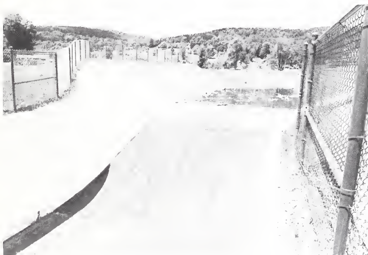
A transition structure was built to smoothly funnel floodwater into the narrow concrete outlet channel.
