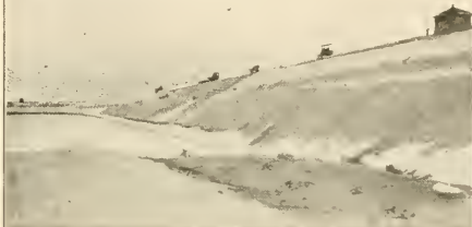
67. "Belle Fourche Irrigation Reservoir," largest earthen embankment in the world 115 feet high, 1 1-8 miles long, faced with concrete blocks, irrigates 100,000 acres, Western South Dakota
