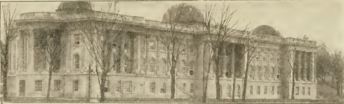
Building Erected at Irvington-on-the-Hudson for The Cosmopolitan Magazine and The Twentieth Century Home
