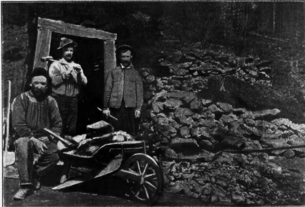
TRAIL CREEK BEGINNINGS, "LILY MAY" TUNNEL.
