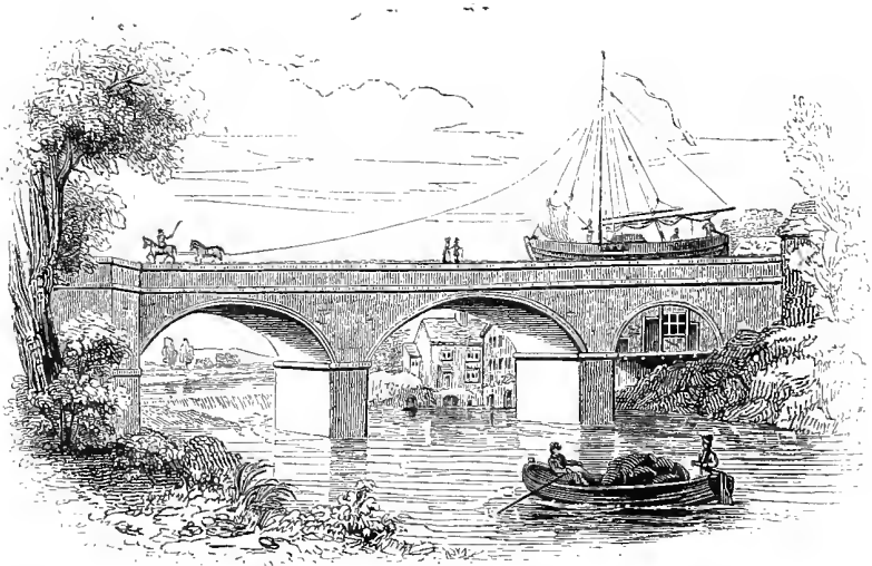
Canal Aqueduct over the Irwell.
