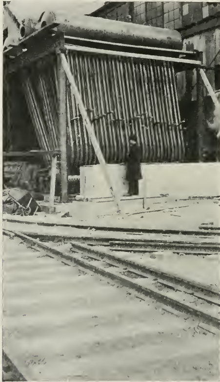
FIG. 12.—One Type of Boiler Used in the New York Tunnel Plants.
