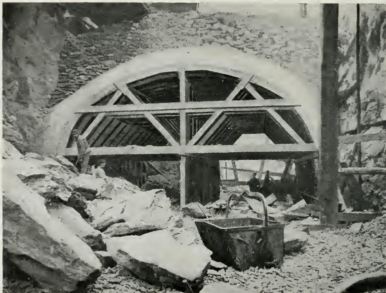
Concrete Arch Subway Construction in Open Cut.
