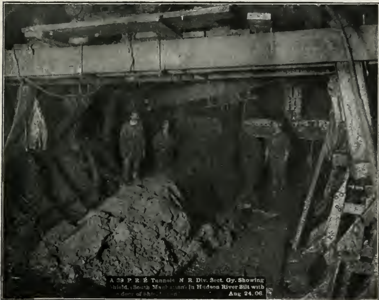
Interior of Shield in P.R.R. North River Tunnel, Showing Silt Entering Through One Open Door.
