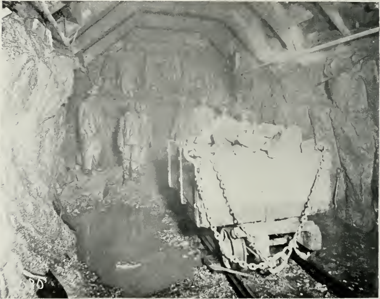
Drilling and Mucking in East River Subway Tunnel.
