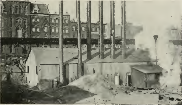
FIG. 1.—Temporary Power House, Pennsylvania Terminal.
