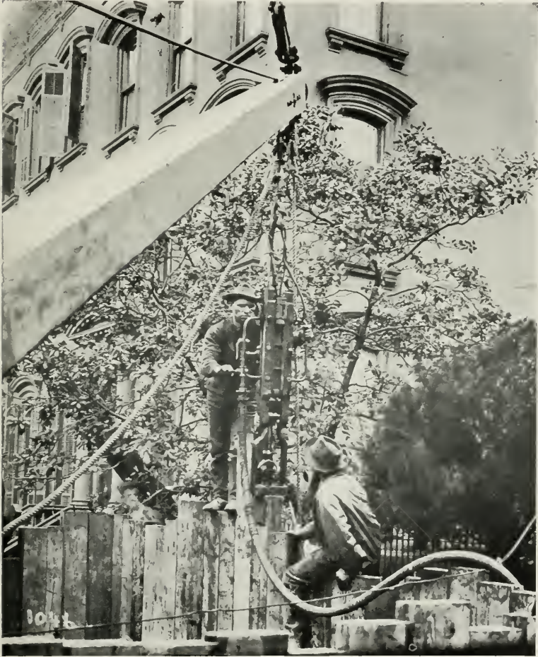
Driving Sheet Piling with an Ingersoll-Rand Sheet Pile Driver on Subway Construction in Brooklyn.
