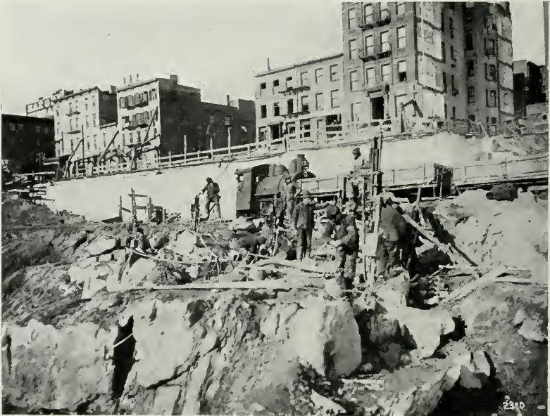
Ingersoll-Rand Rock Drills in P. R. R. Terminal Excavation.
