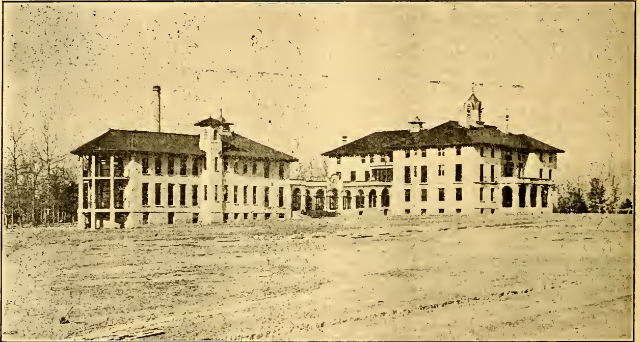
THE NEW WATTS HOSPITAL RECENTLY COMPLETED AT DURHAM.
