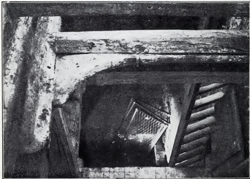
Fig. 1.—CELLAR OF No. 6, HIGH STREET.
