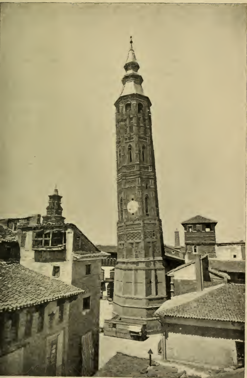
THE LEANING TOWER AT ZARAGOZA.
