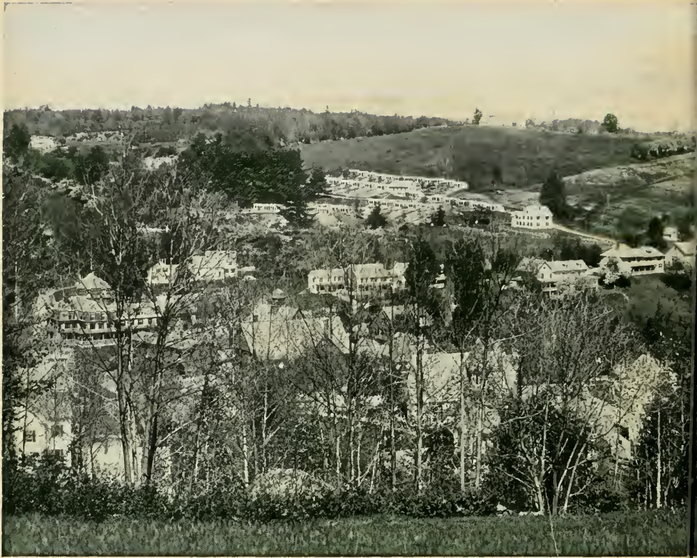
GENERAL VIEW OF NEW BOSTON AND VALLEY FORGE
