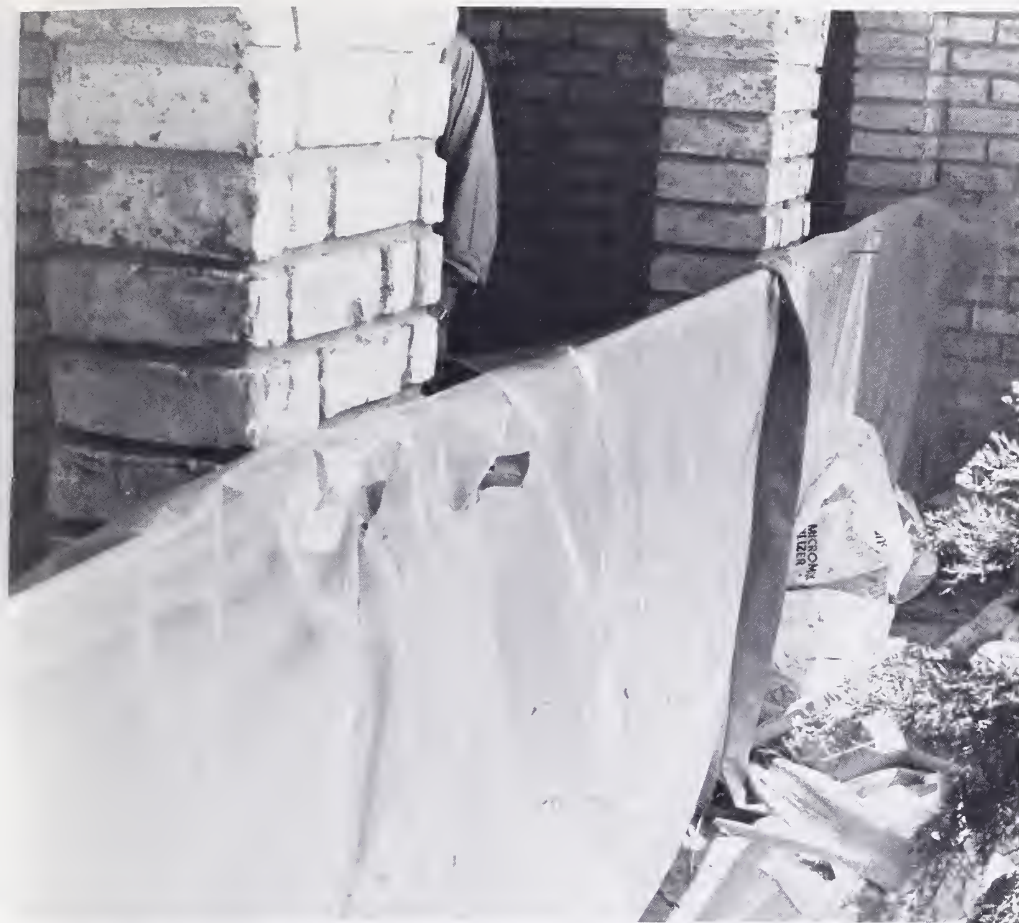
Three 100-foot rolls of polyethylene plastic sheeting wrapped the McManus home against floods that ravaged southeast Louisiana earlier this year.
