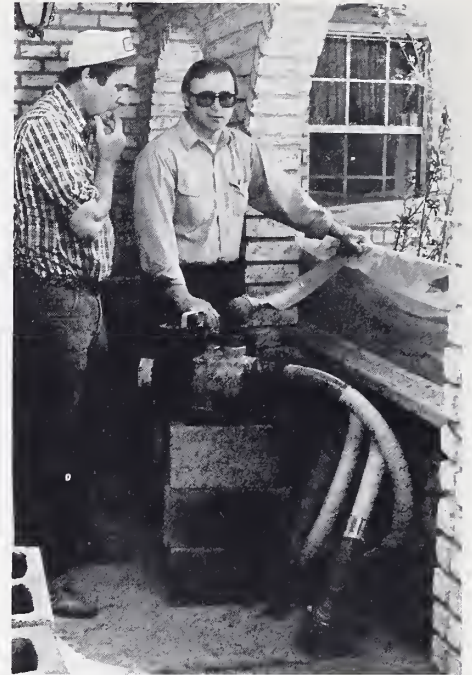
When the floods came they were ready! Extension agricultural engineering specialists Ray McManus (left) and Gene Baker check out the gasoline-driven sump pump that operated from behind a water-tight barrier and kept rising floodwaters to a minimum.
