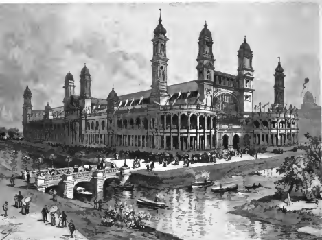
THE ELECTRICAL BUILDING.
