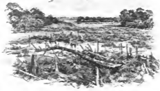
CANAL CLEARING, LOOKING WESTWARD ACROSS LAJUNA DESAHO.
