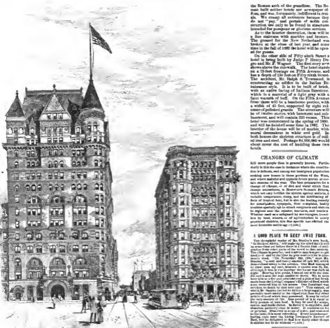
THE TWO NEW HOTELS AS THEY WILL STAND AT FIFTH AVENUE AND FIFTY-SIXTH STREET, NEW YORK.
