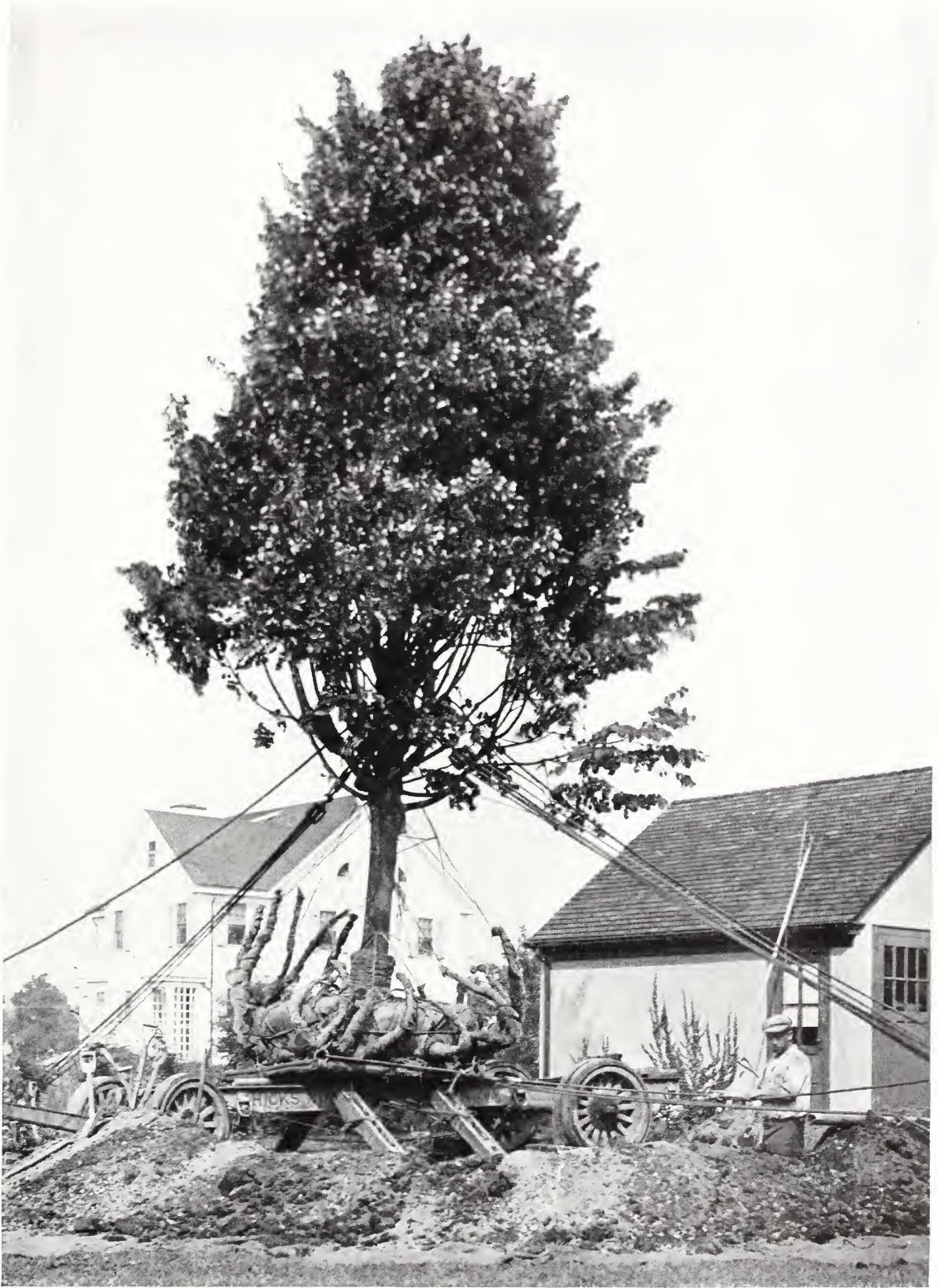
This shows a large Linden tree from our Nurseries being planted last summer, in full leaf, at residence in Garden City. Note the large ball with extending roots carefully wrapped. Such planting in summer is not an experiment; we have been doing it many years and guarantee successful results.
