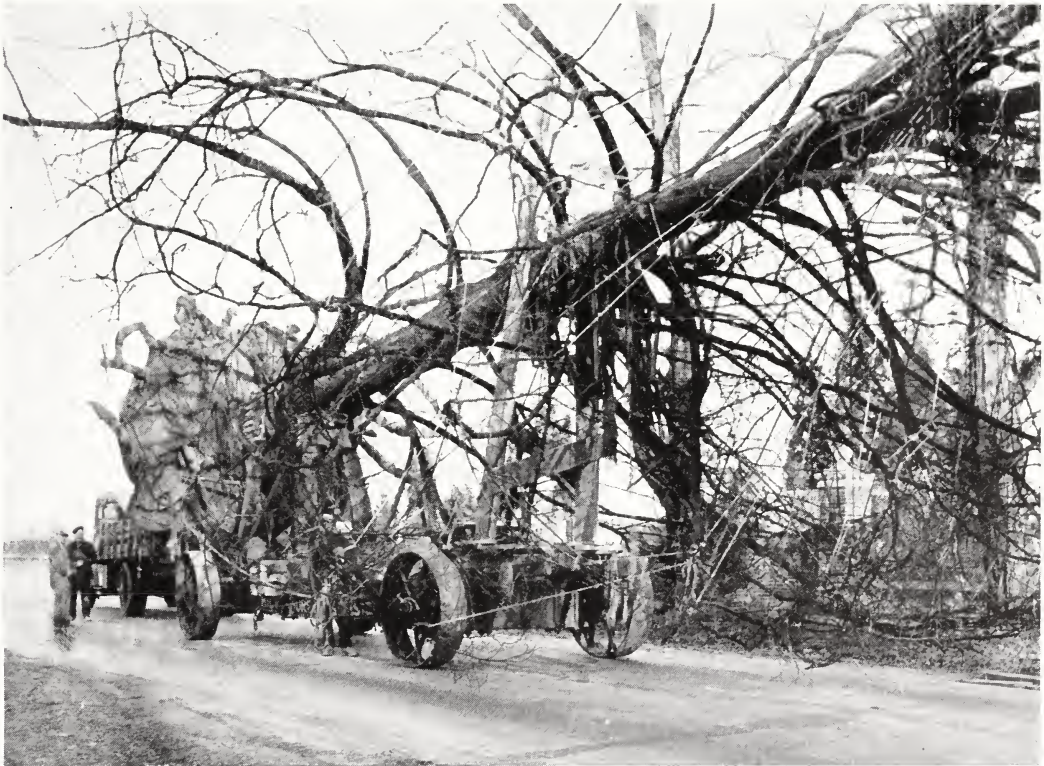
Large Linden being moved to estate of Mr. Marshall Field, Huntington, L. I. Two such trees were successfully transplanted. Note the Hicks' way of digging with large balls of earth and saving all extending roots by carefully wrapping, to prevent drying out.
