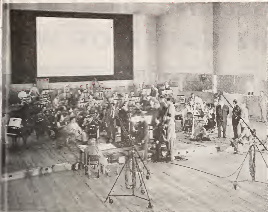
THE WORLD'S LARGEST recording stage is the one above, at the Republic Studio. It is one unit of a $2,000,000 1945 expansion program. The scoring stage is 120 feet long, 75 feet wide and 32 feet high; its volume is 250,000 cubic feet. The building contains a separate vocal room, an adjustable reverberation chamber, and projection rooms.
