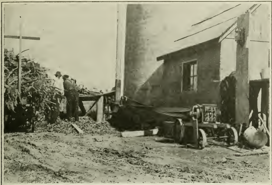
Blower Type of Ensilage Cutter
