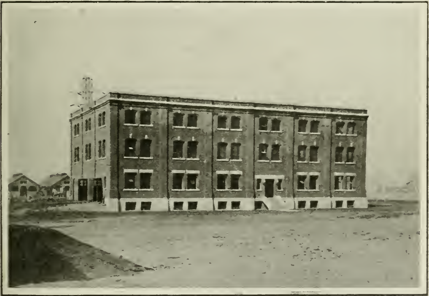
Toronto Laboratory and Storehouse
