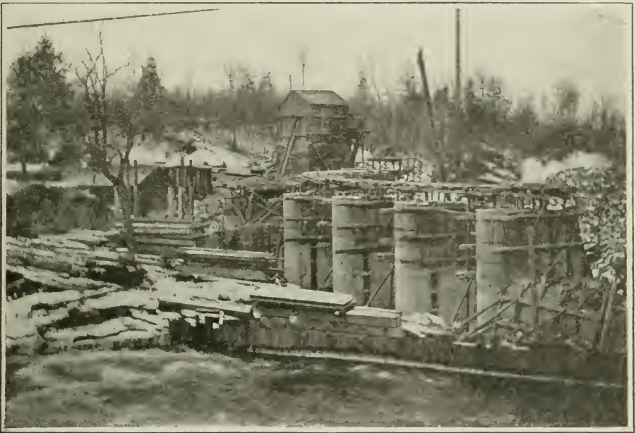
Wasdell's Falls Construction—Completed Piers—Main Dam.
