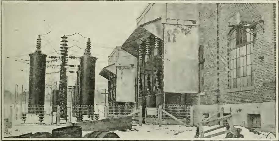
Niagara Falls Transformer Station, 110,000 Volt Arresters and Outdoor Switches
