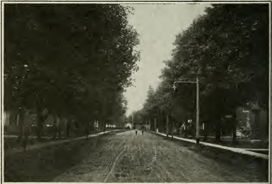
Lighting in Residential District, Galt
