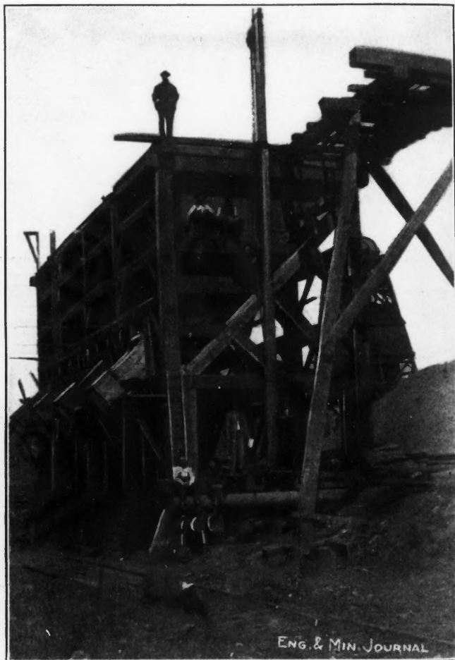
ORE DOCK FOR LOADING INTO RAILROAD CARS. OLD WOODEN TYPE, SEPARATE FROM SHAFT HOUSE
