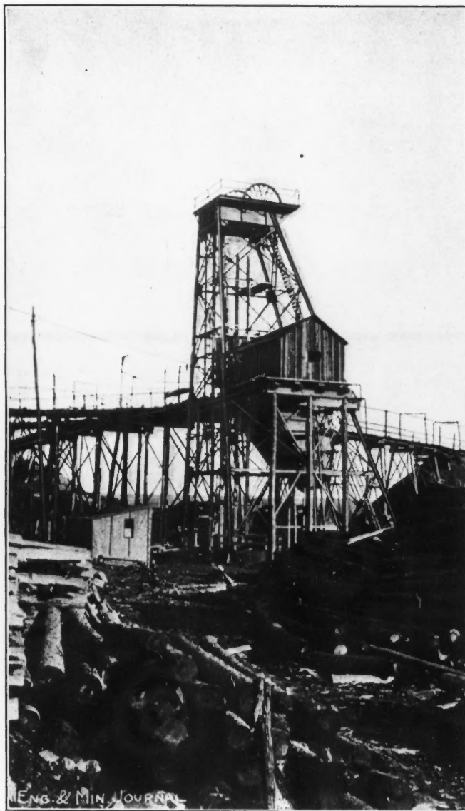
STEEL HEADFRAME OF VOLUNTEER MINE OF VOLUNTEER ORE CO.
