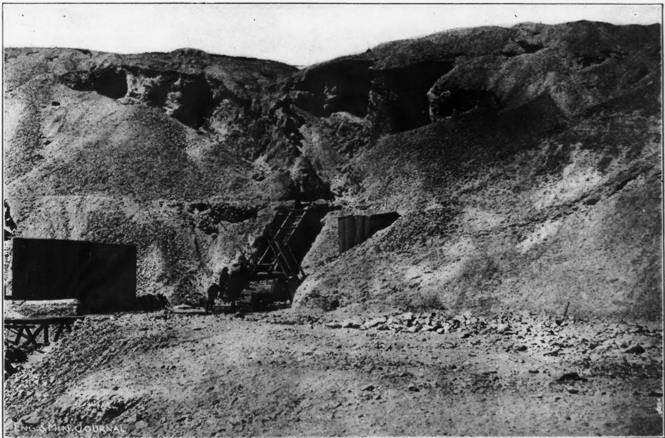
THE CONSTANCIA OPENCUT AND OLD SCREENING PLANT
