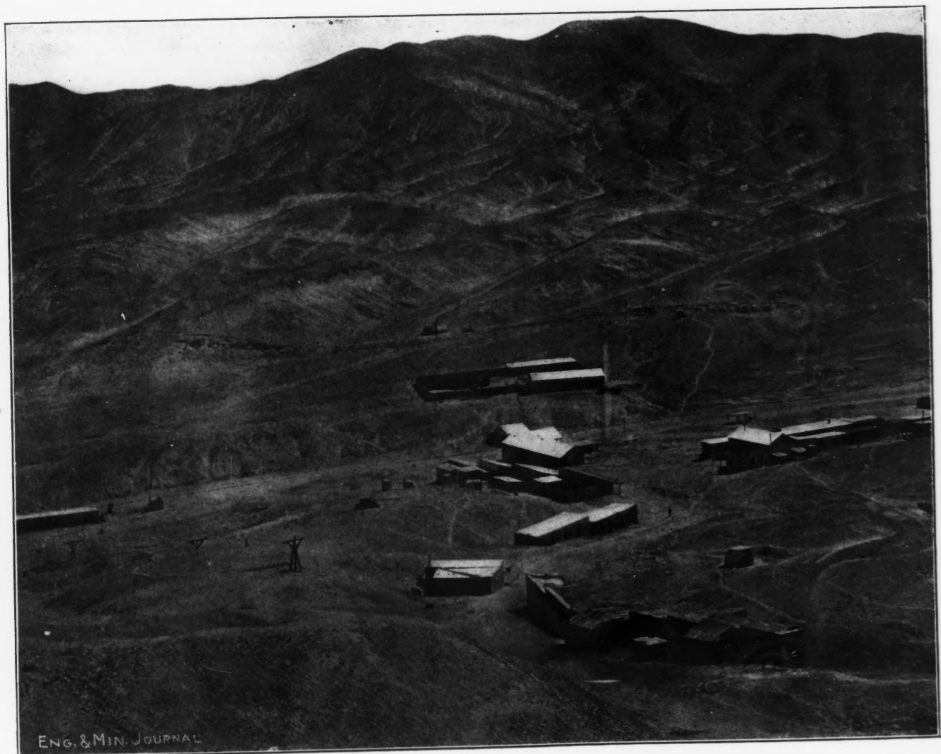
THE OLD CAMP AT THE MINE. NOW BEING REBUILT
