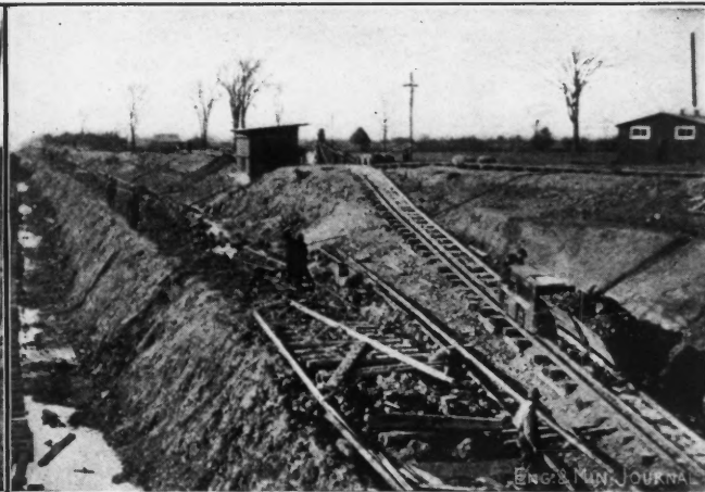
HAULING 6-TON LOAD UP 12½% GRADE
