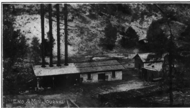
FIG. 1. DURAZNO POWER PLANT
