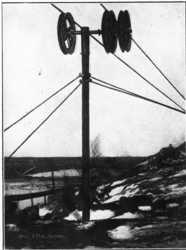
PULLEY STAND OF PIPE GUYED WITH OLD CABLE
