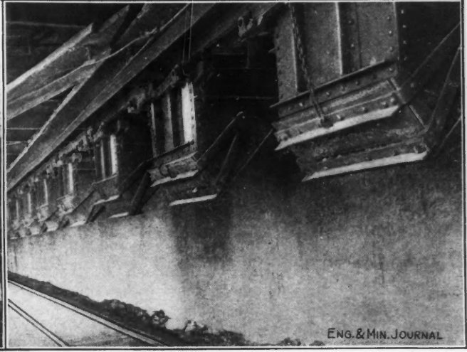
WEIGHING HOPPERS UNDER STOCK BINS
