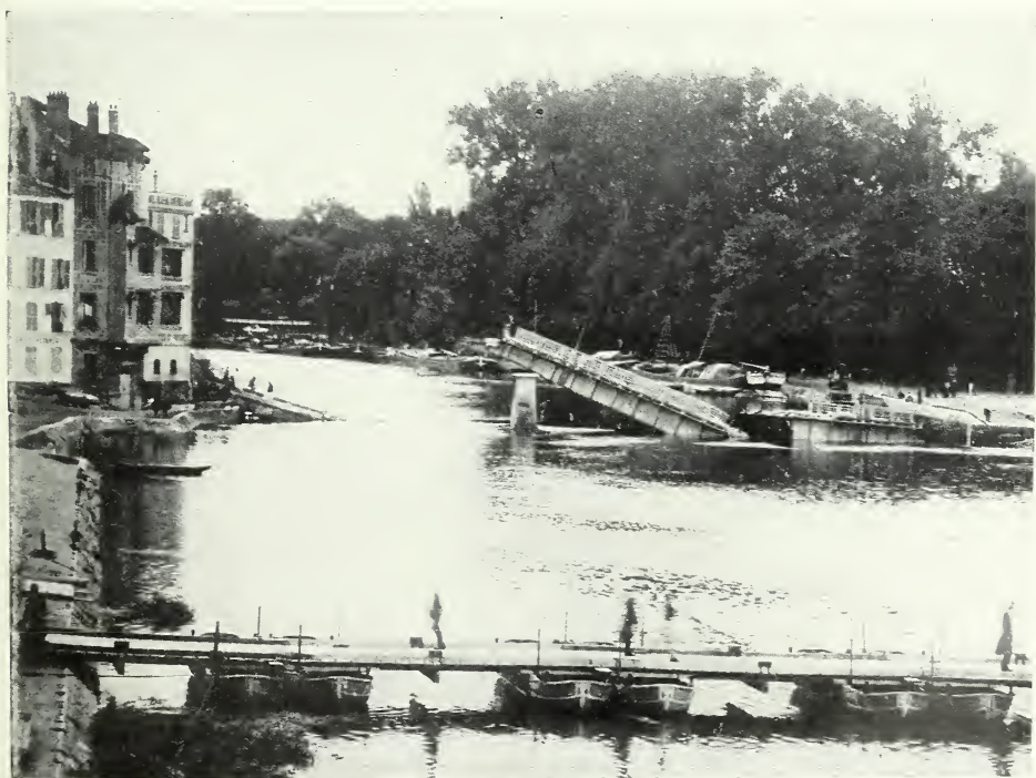
Bridge at Lagny destroyed by the British forces in their retreat before the Germans and pontoon bridge built to pursue the latter on their retreat during the Battle of the Marne.
