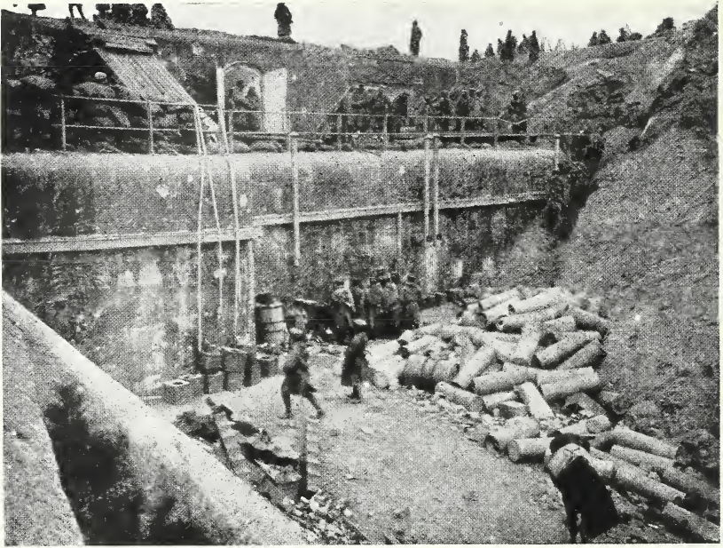
Fort Iltis, at Tsing-Tau.
