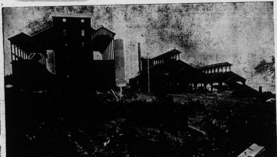
VIEW FROM REAR OF SMELTER LOOKING SEAWARD.
