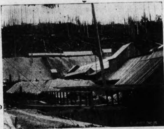
DUMP OF LENORA MINE, MT. SICKER.
