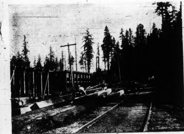
TYEE ORE BINS, LADYSMITH, CAPACITY 1000 TONS.
