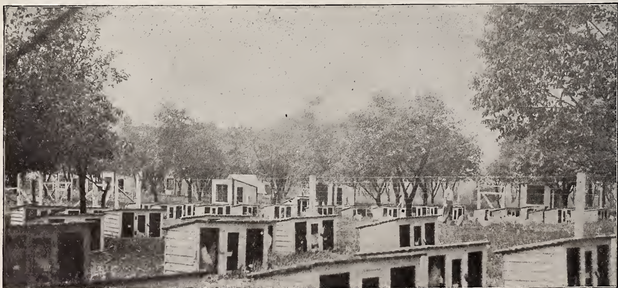
In the above illustration may be seen a portion of the cockerel and colony houses at the Aldrich Poultry Farm, Columbus, Ohio. The advantages of the colony house system of growing young stock is fully appreciated by every practical poultry raiser, as it has been demonstrated that this method produces birds that excel in health and vigor and is a material aid to quick maturity.
