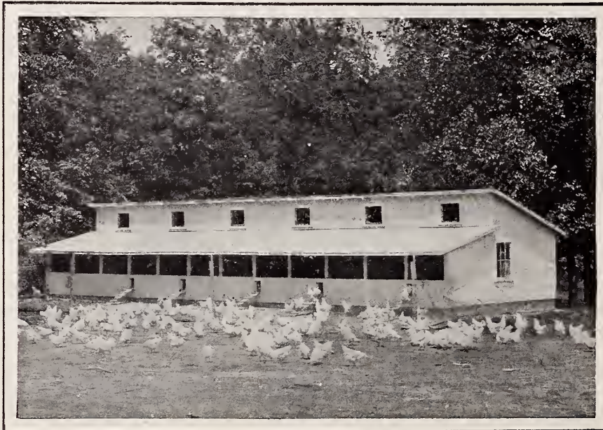
We seldom see a more desirable location for a poultry house than the one illustrated above, both range and shade are plentifully supplied. The house in the picture is one of four new ones recently erected by U. R. Fishel, Hope, Indiana, and it indicates the rapid progress that is being made at Fishelton.
