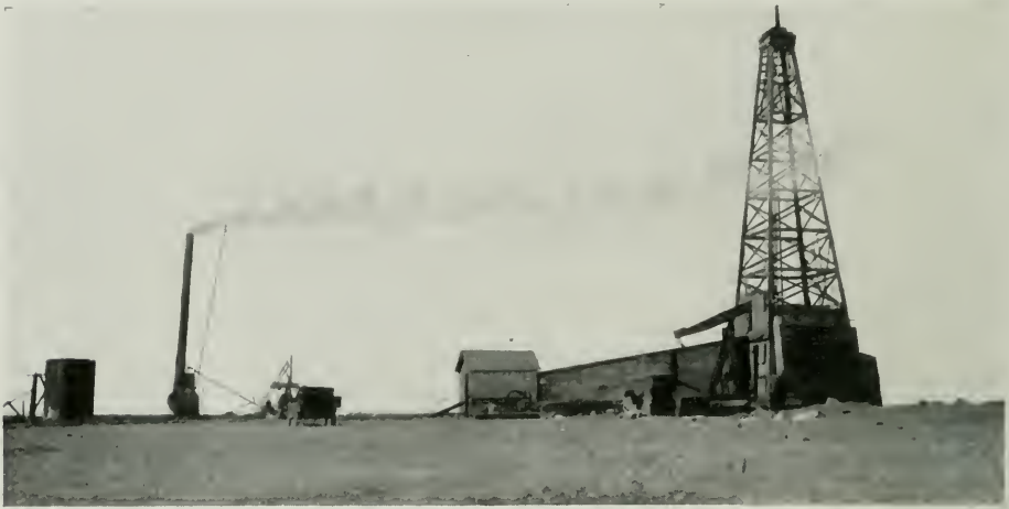
Drilling a gas well.
