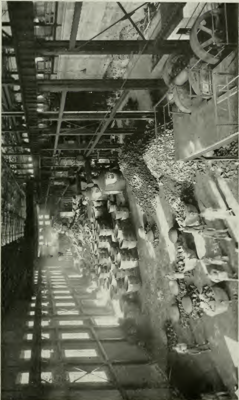
International Nickel Company of Canada, Port Colborne—Bird's-eye view of casting room.
