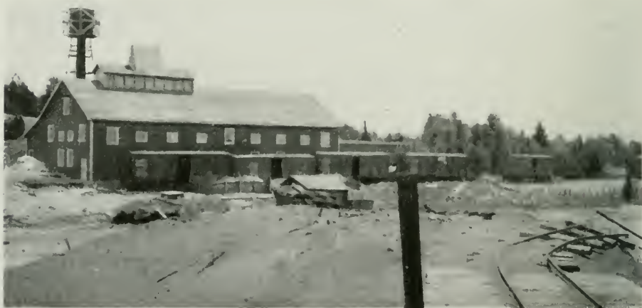
Electric furnace for producing ferro-chrome, Cordova Mines.
