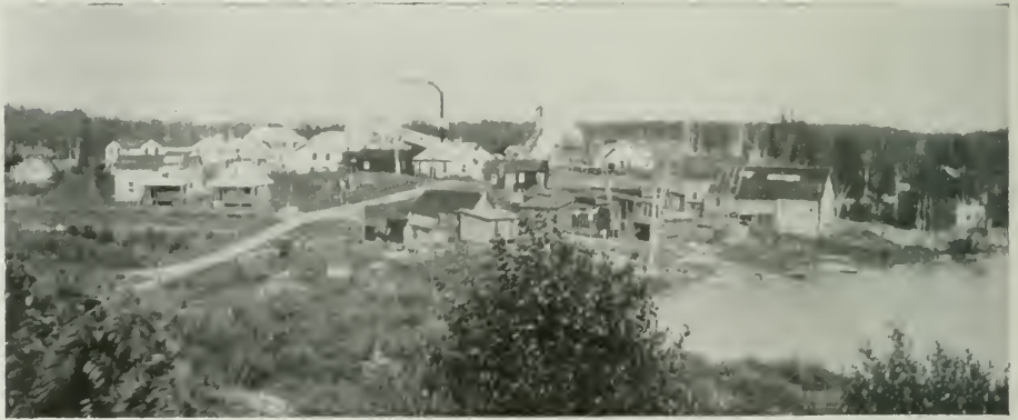
Teek-Hughes mine, June, 1919. The two buildings with verandahs in the foreground on the left belong to the Kirkland-Porphyr.
