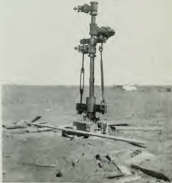
Gas well after derrick is removed. Ready to turn into the line.
