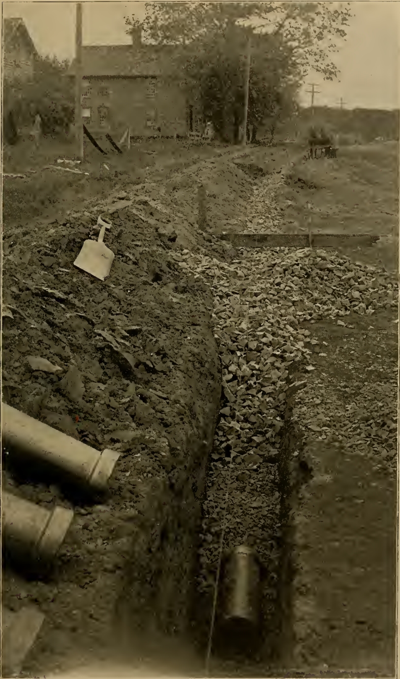
WESTFIELD ROAD, MASS., 1894. View showing details of drain.
