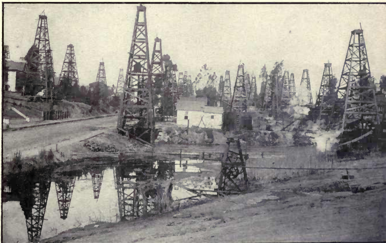
FIG. 2.— View in Los Angeles, Calif., oil field. Such close spacing of oil derricks tends to hasten the exhaustion of the oil supply.
