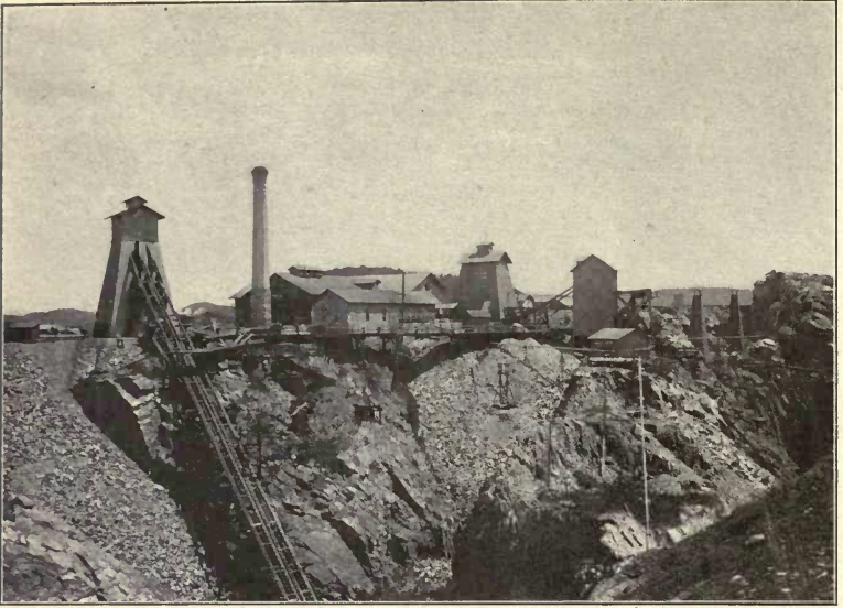
FIG. 1. — Iron mine, Soudan, Minn. Shows old open pit with jasper horse in middle.
