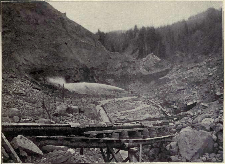
FIG. 1.—Hydraulic mining of auriferous gravel. The sluice box in the foreground is for catching the gold.
