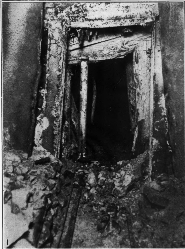
TREATED AND UNPROTECTED TIMBERS AT NORTH BUTTE MINE
