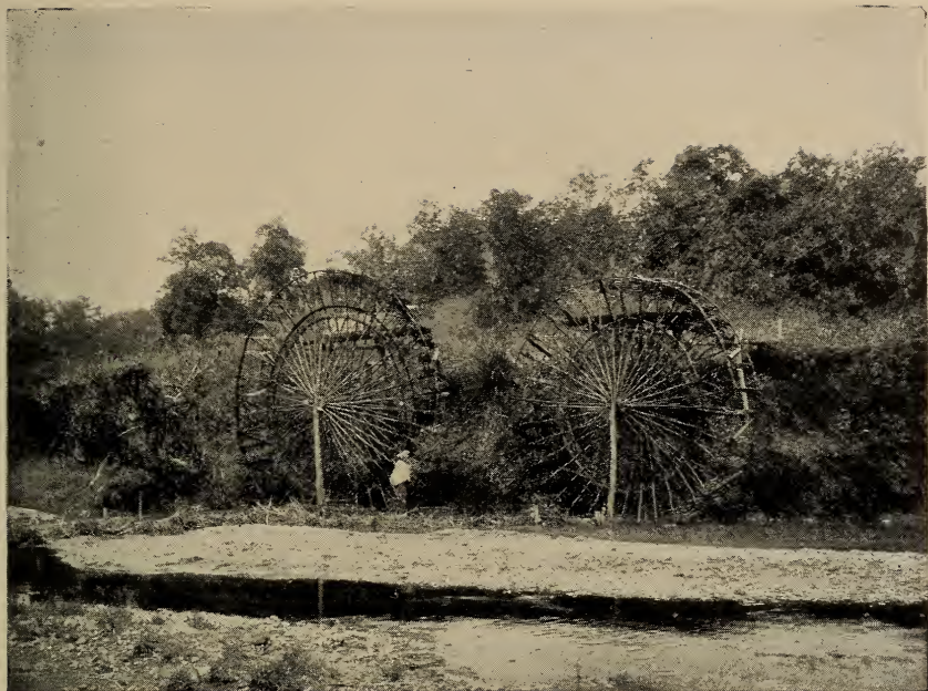
NATIVE IRRIGATION WHEELS. (Rattan wheels, wattle paddles, bamboo buckets, wooden pipes.)
