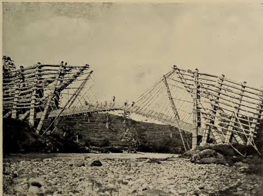
NATIVE ENGINEERING : A BAMBOO CANTILEVER BRIDGE.
