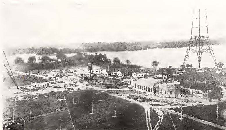
U. S. NAVAL HIGH POWER RADIO STATION
