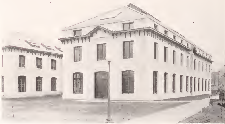
EXTENSION TO ISHERWOOD HALL
