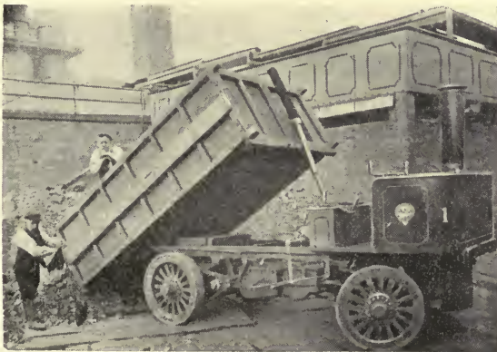
Fig. 70. Telescopic-Screw Tipping Gear.
