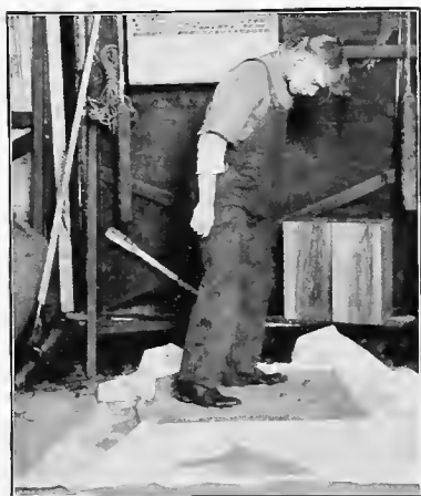
Packing the top layer of Sawdust. The Sawdust should be warm and packed down carefully.
