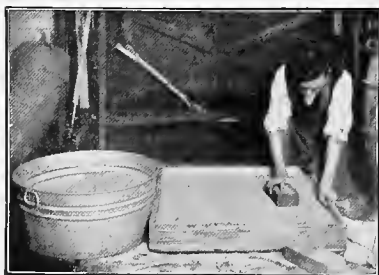
Packing Sawdust in Germinating Box. A Brick is convenient for this. The Surface should be left even and smooth.
