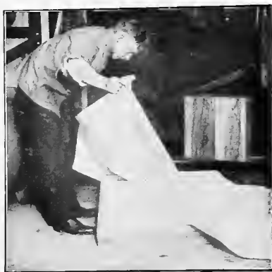
Laying on the outside Top Cloth.
