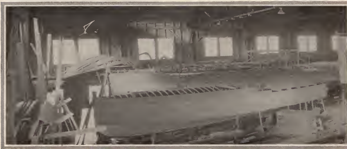
An interior view of the finishing plant showing
