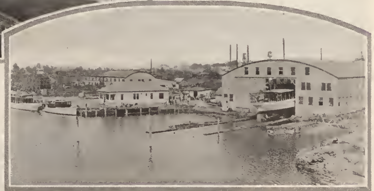
Just before the launching of the steel Diesel yacht Sylvia in June
