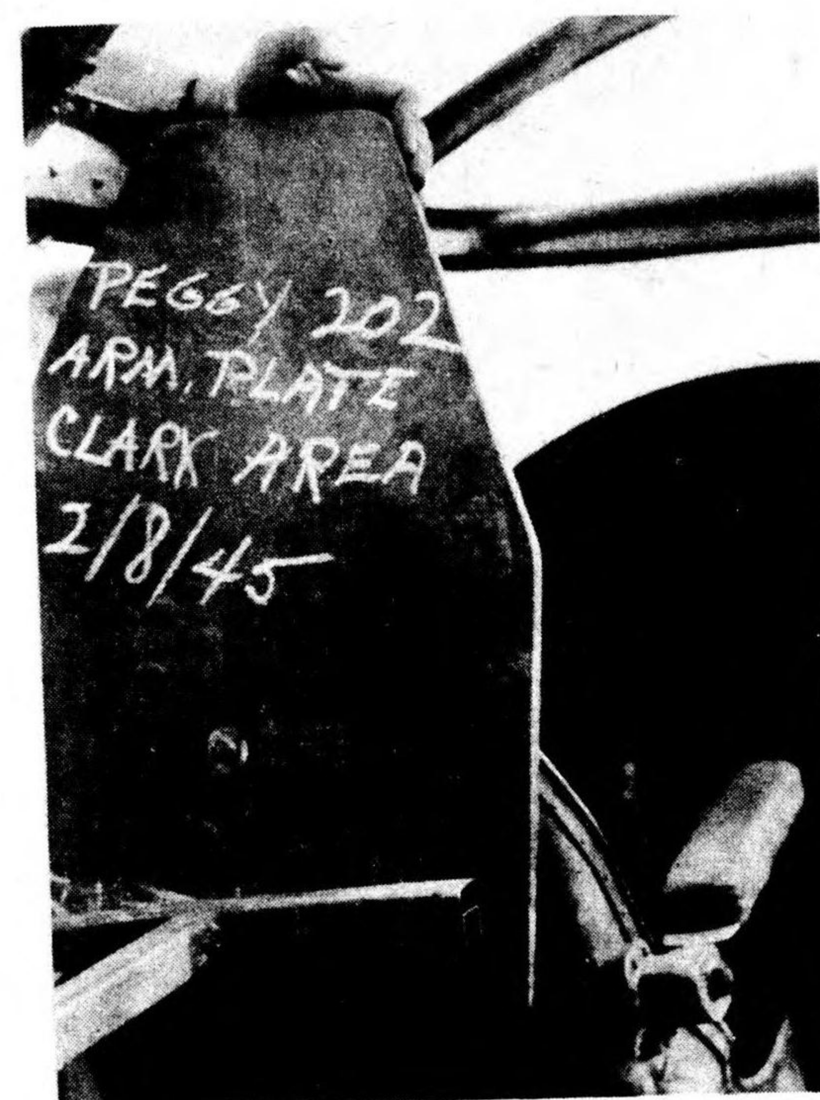
Figure 23 Armor plate for pilot's seat
