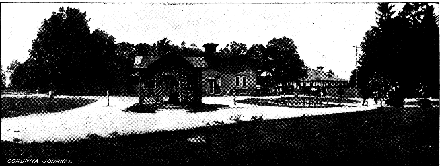
Residence of Hugh McCurdy. Casino in the Distance
