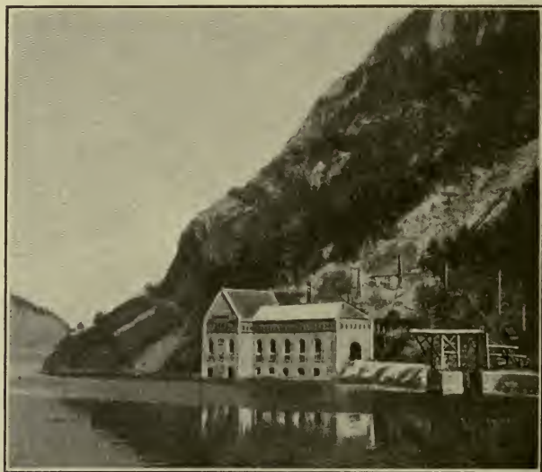
FIG. 33.—View of the Tyselfaldene Power House. 1
