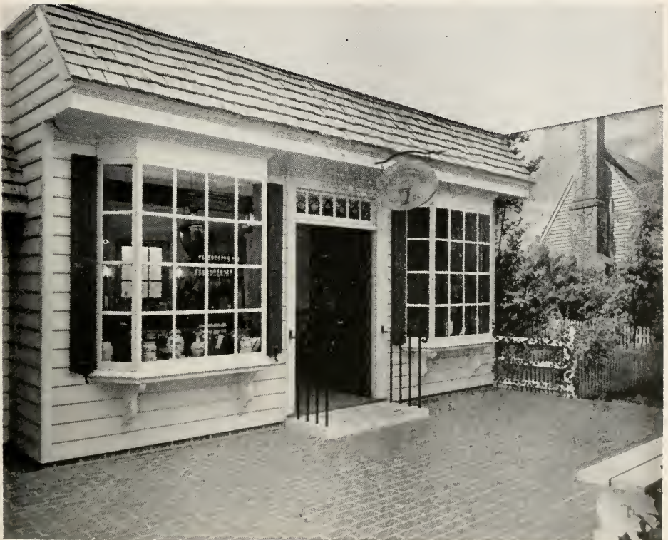
The exterior view of the Lederle Old Apothecary Shop shows the mural, the brick, paving, the iron cleats in the steps, old "bullseye" glass above the door, hand split shingles, and other details of construction.
