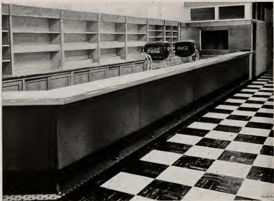
A recent installation of Bastian-Blessing Soda Fountain equipment in the Student Union Building, East Carolina College, Greenville, North Carolina.
