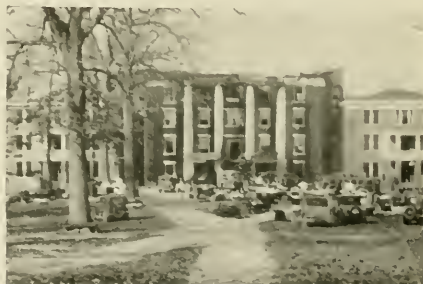
Main Building Damaged by Fire 1928
