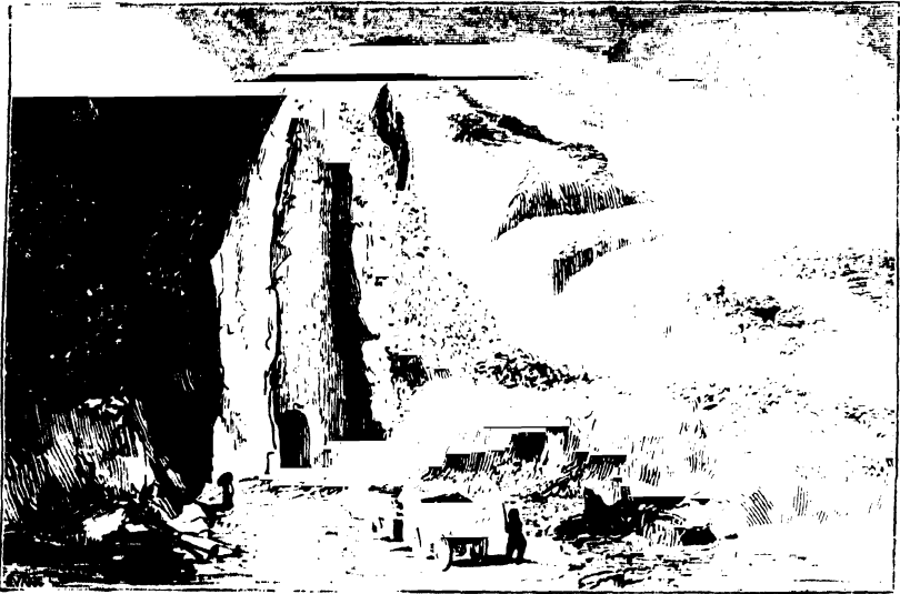
Entrance to Odin's Mine.
