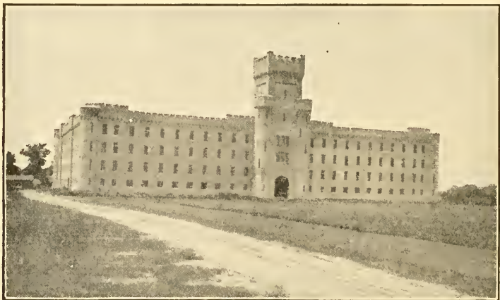
BARRACKS BUILDING ON THE NEW SITE OF THE CITADEL IN CHARLESTON.
