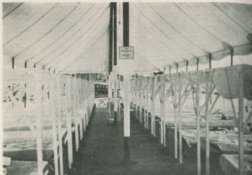
INTERIOR OF WARD TENT.
