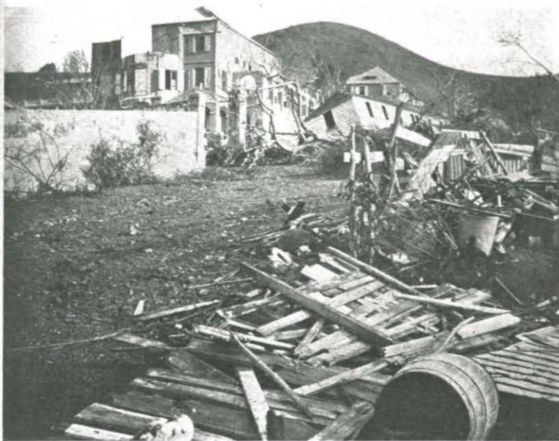
HOSPITAL AT CHRISTIANSTED AFTER THE HURRICANE OF OCTOBER, 1916.
