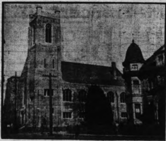
With the completion of the tower of the First Presbyterian church, one of the finest church towers in Victoria has been finished in the ecclesiastical centre of the city. The picture is taken from Quadra street frontage.
