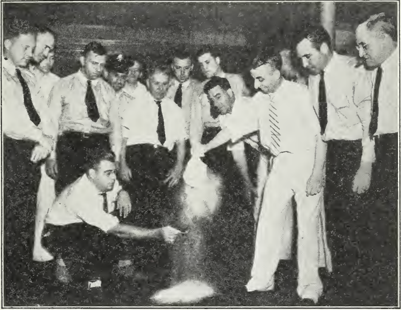
FIGURE 10.—Demonstration of explosibility of dust at Virginia Firemen's Training School, Richmond, Va.
