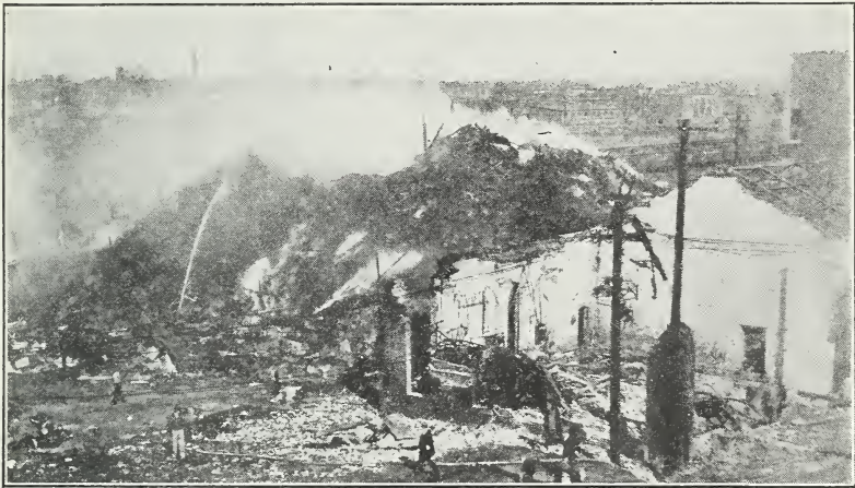
FIGURE 1.—After an explosion in a terminal grain elevator. Four men were killed in this explosion.
