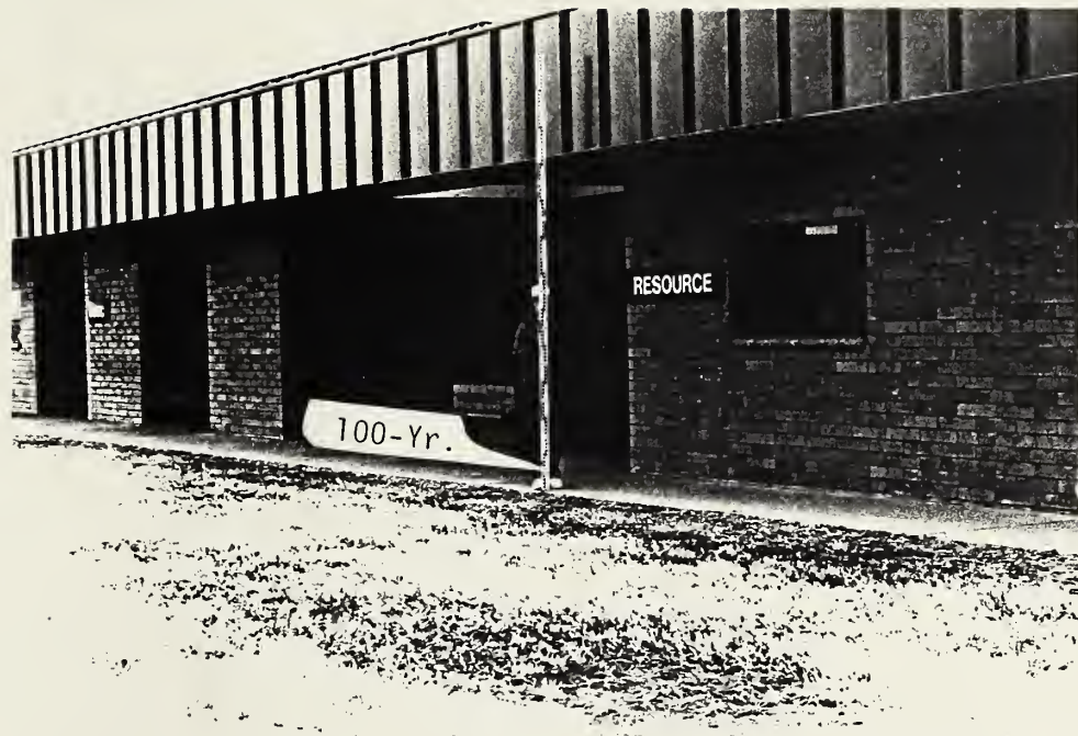
Special Education and 5th Grade Building, Palominas School Complex, looking northeast. Depth, 0.5 ft.
