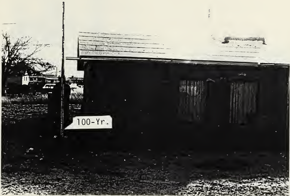
Along Healing Way Road between Second and Third Avenue looking east. Depth, 1.0 ft.
