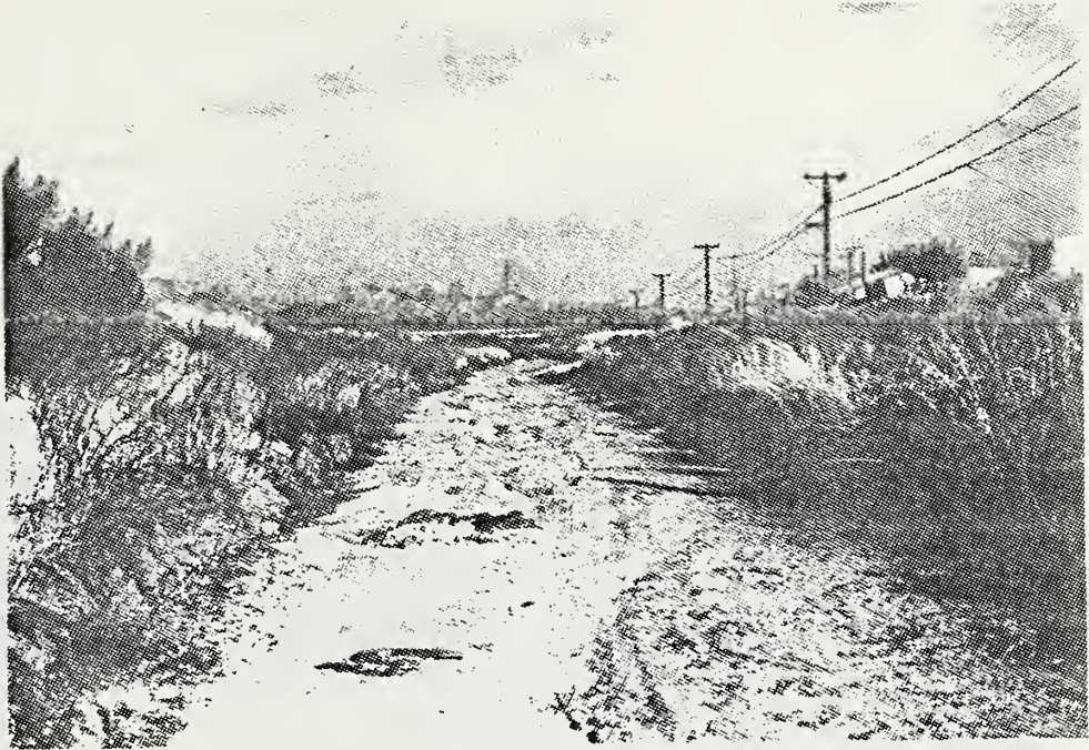
Figure 4 School House Wash near Loaves and Fishes Drive Maximum Capacity about 1900 cfs
