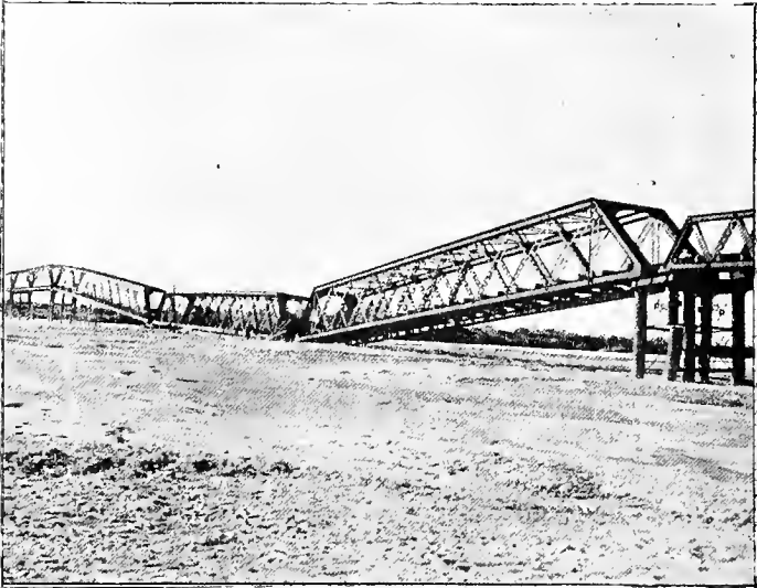
NAGARAWA BRIDGE AFTER THE EARTHQUAKE.
