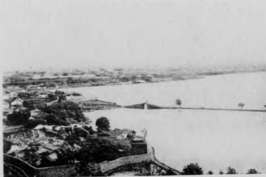
(11) Distant View of the "Broken-off" Bridge
