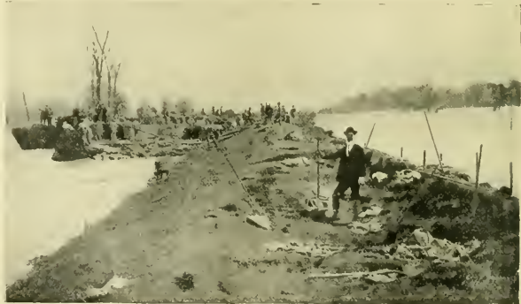
FIG. 2.—Repairing levee at Lagrange, Mississippi.
