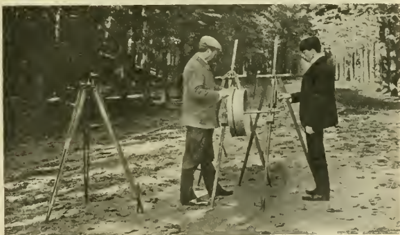
FIG. 5.—Rolling of a 2 km. wire on an aluminium drum.
