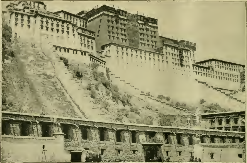
FIG. 1.—Part of the Potala Palace from the buildings at its base. It is built of granite and whitewashed once a year. The dark central portion is crimson. From Landon's "Lhasa."
