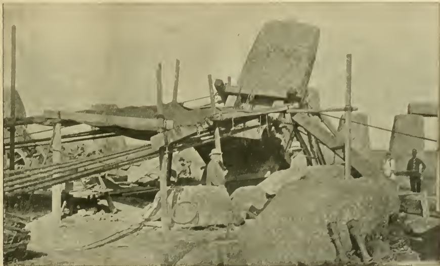
FIG. 4. The arrangements for raising the stone.
