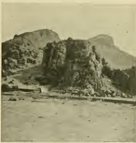
FIG. 1.—Cliff showing columnar structure of iron-ore at western end of the Cerro Mercado or Iron Mountain of Durango, Mexico.
