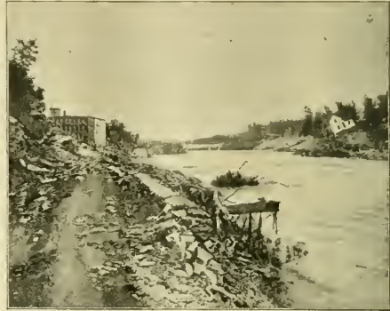
FIG. 2.—Clifton after the flood of 1903.
