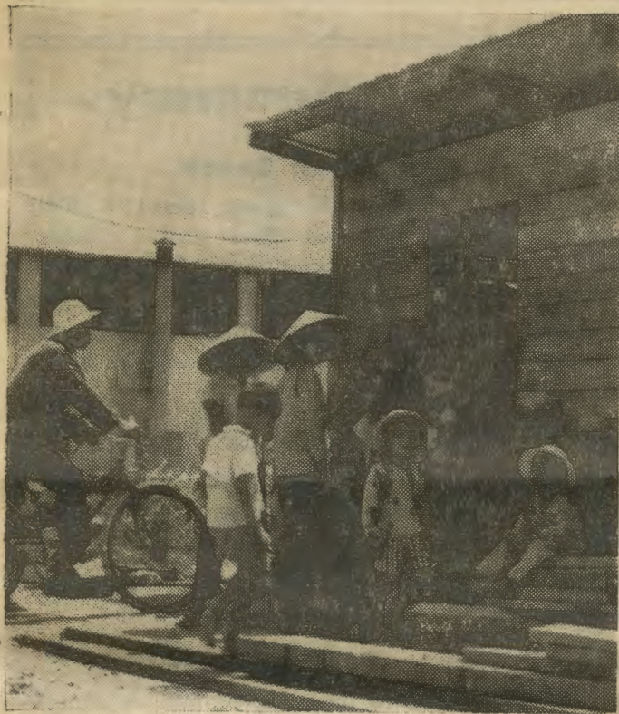
NEW HOME — Vietnamese family at Hoa Buong prepares to move into home built by Seabees. Lumber in front of house will furnish home's interior. (USN Photo)
